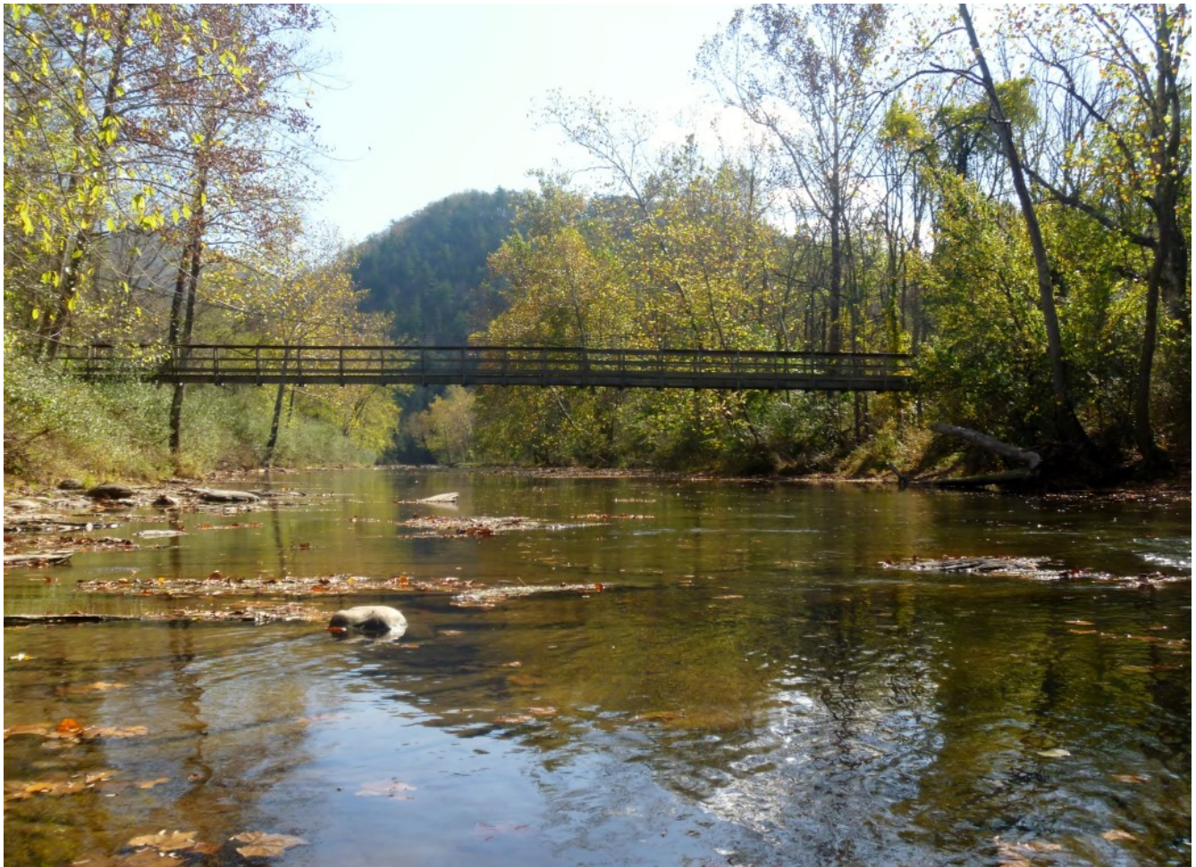
The Cowpasture River Lazily Flowing Through the U.S. Forest Service Wallace Tract in the Fall This Swinging Bridge Demonstrates Classic Wooden Bridge Towers, Deck and Rails Photographic Attribution Hereby Given to C. Nelson Hoy
