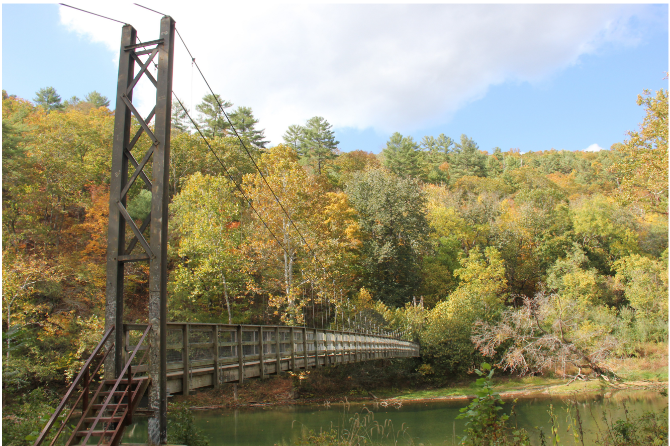
USFS GWNF Warm Springs Ranger District, Walton Tract Swinging Bridge Photographic Attribution Hereby Given to Kathy Farmer
