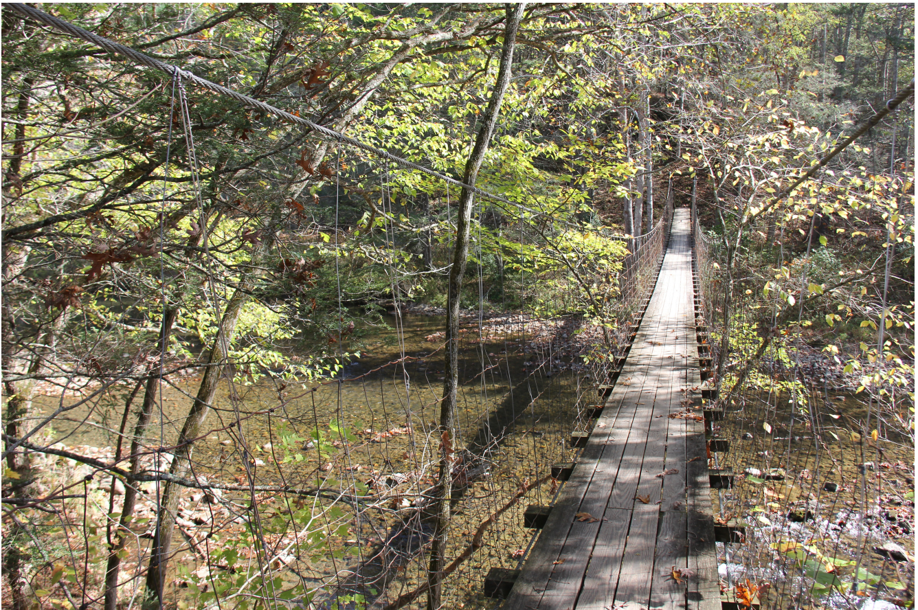
Bullpasture River Gorge Swinging Bridge Owned and Operated by the VDGIF Highland Wildlife Management Area Photographic Attribution Hereby Given to Kathy Farmer
