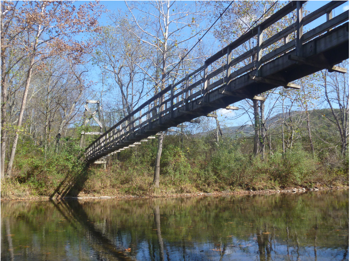
USFS GWNF North River Ranger District, Wallace Tract Swinging Bridge Demonstrating Classic Wooden Bridge Towers, Deck and Rails Photographic Attribution Hereby Given to C. Nelson Hoy
